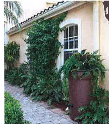
A rain barrel captures and stores roof runoff for later use. A planter incorporated as the top of the rain barrel provides camouflage.
