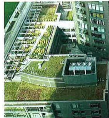
A green roof absorbs rainwater, reduces energy costs and offers wildlife habitat in urban Portland, Oregon.
