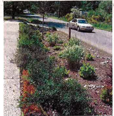
A roadside swale built in a public right-of-way provides aesthetic benefits and collects and filters road runoff in Olympia, Washington.
