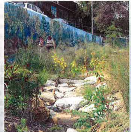
An open space next to a school in Philadelphia was transformed into an outdoor learning lab, recreation area and stormwater management system (rain garden) that captures and filters parking lot runoff.
