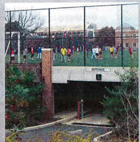
The roof of this Washington, D.C. parking garage doubles as a school athletic field, reducing runoff and offering usable open space.
